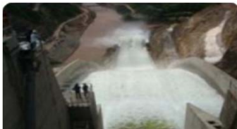
Hydro - Tehri 1,000 MW - India
